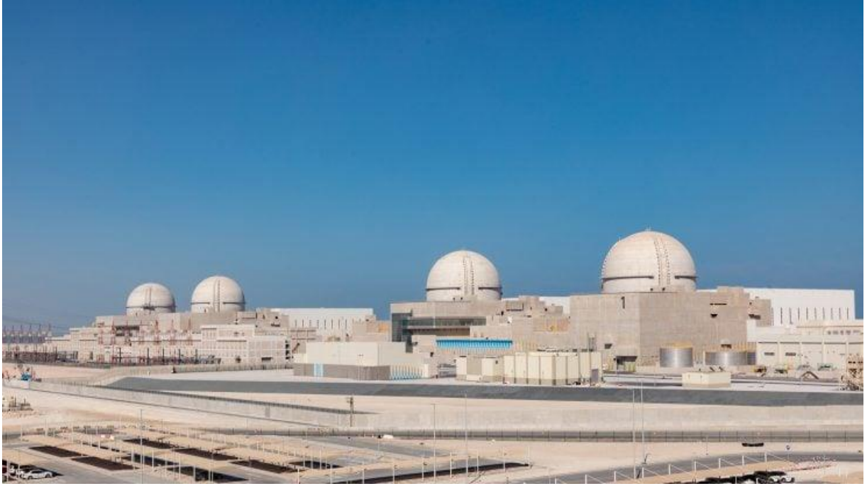
Kaynak: Emirates Water and Electricity Company – EWEC
